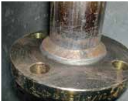
Small bore pipe to flange weld
