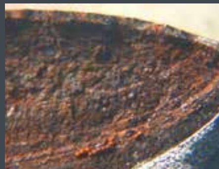
A fatigue crack propagating top to bottom through the pipe
