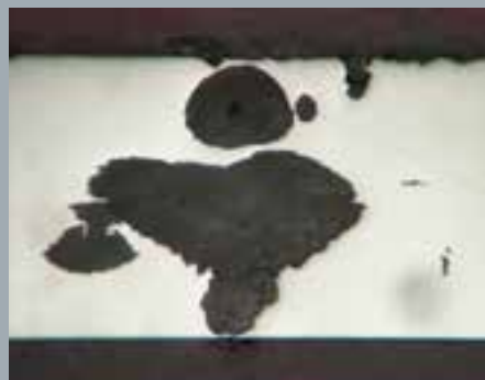
Cross section through pinhole revealing large underlying corrosion pits
